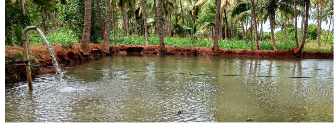
Farm Pond constructed under the project (Source: RTI International)
