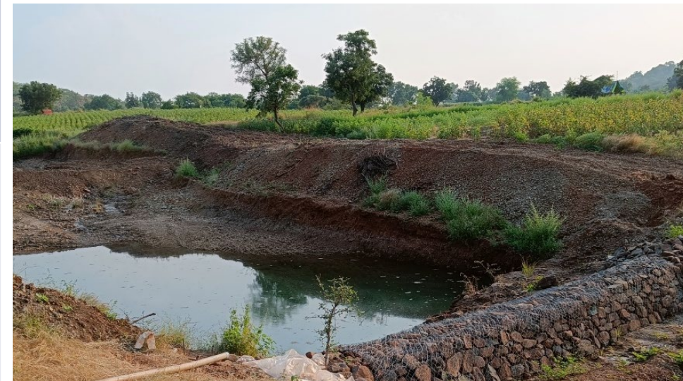
Gabion structure that was constructed (Source: RTI International)
