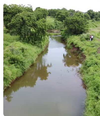
Nala deepening at Jalgaon along with well recharge
